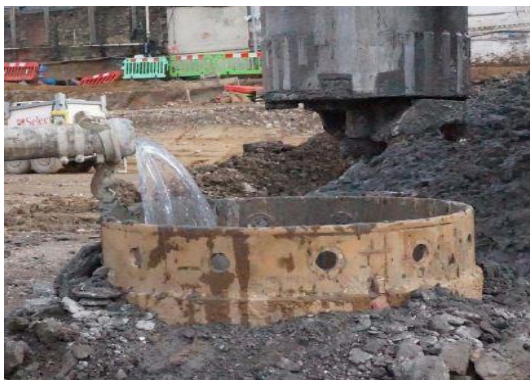
Polymer Slurry being pumped into borehole through a Diaphragm Pump
